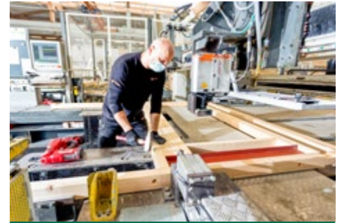
assembly of the wooden framework by workers
