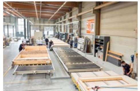
fast handover of the paneled house walls for the next production stage
